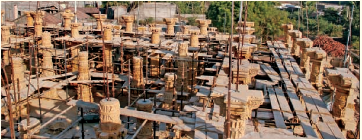
Copper rods inserted through the pillars as part of the mandir's earthquake-resistant structural design
