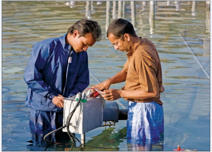
Volunteers checking the electrical installations
